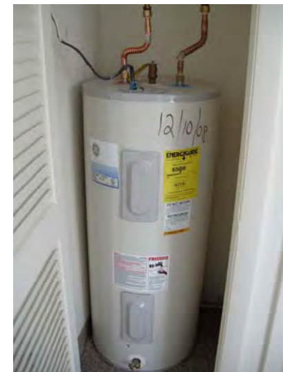
Typical dwelling unit domestic hot water heater
