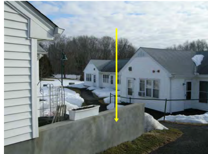
Typical poured concrete retaining wall at grade change
